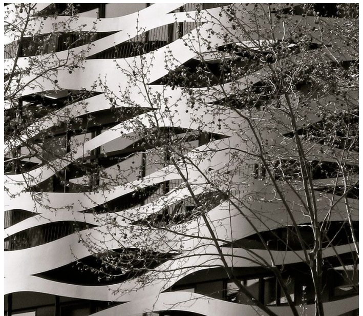
Façade renovation of Suites Avenue Aparthotel (Figure.9)
