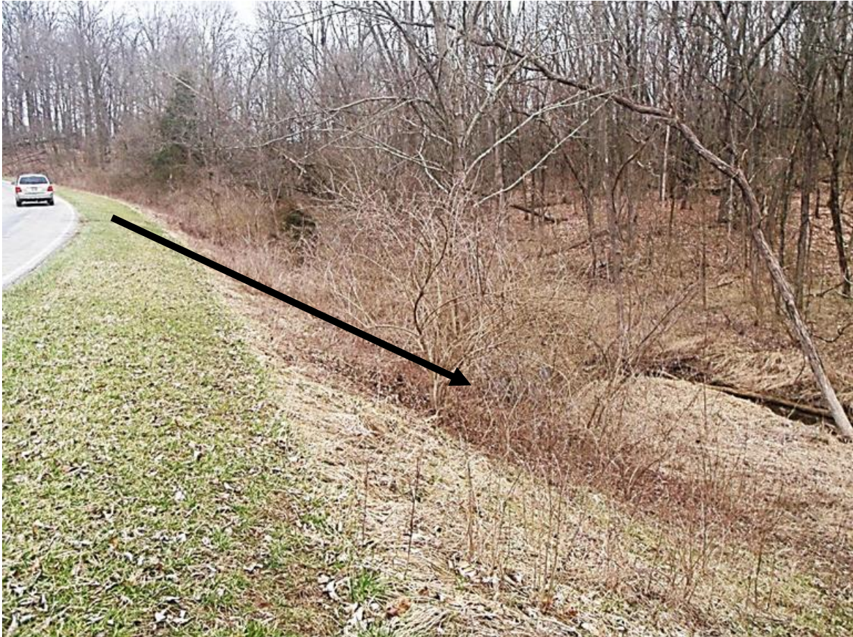
FIGURE 5 ROADSIDE SLOPE ALONG MAIN LOOP ROAD AT HWSP
